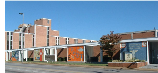
Main Campus - 3rd Street
